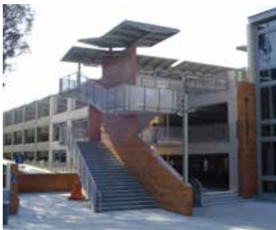
Solar panels on top of parking structure
