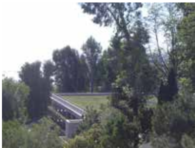
Green roof of a parking structure
