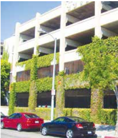
Landscaping softens the appearance of parking structures
