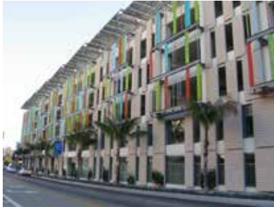
Façade treatments on parking structures provide visual interest
