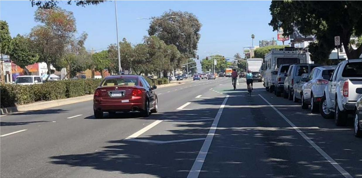
Buffered bike lanes are a type of Class II bike lane in that they are not physically separated from traffic, but are instead given a wide buffer of cross-painted lanes. Parts of Venice Blvd. currently use this setup. The configuration currently consists of two vehicular lanes of traffic, a buffer zone, a Class II bike lane, and curbside parallel parking.
