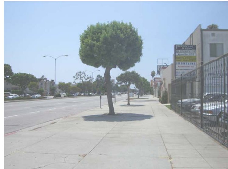
EXISTING SIDEWALK along Venice Boulevard with its vast expanse of concrete sidewalk paving
