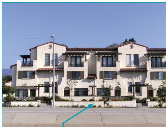
✓ Strong façade rhythm along street frontage is accomplished through the use of architectural elements
