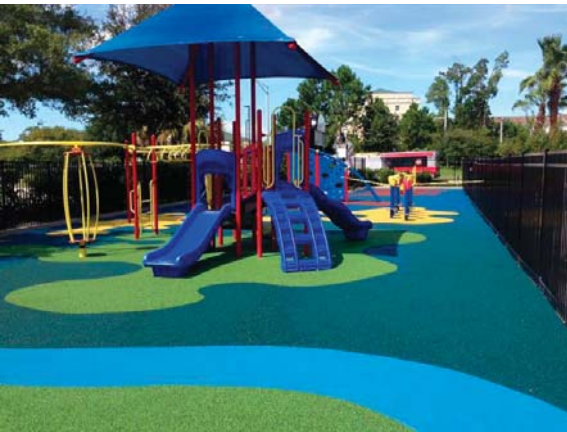
PLAYGROUND: RUBBER SURFACING- POURED IN PLACE
