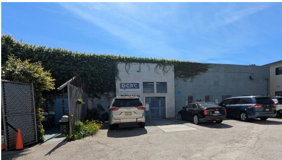
Rear elevation and parking lot. ICF, 2026
